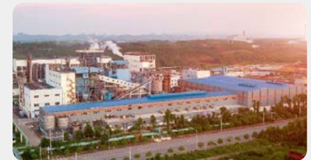
Guangxi YUTO plant
