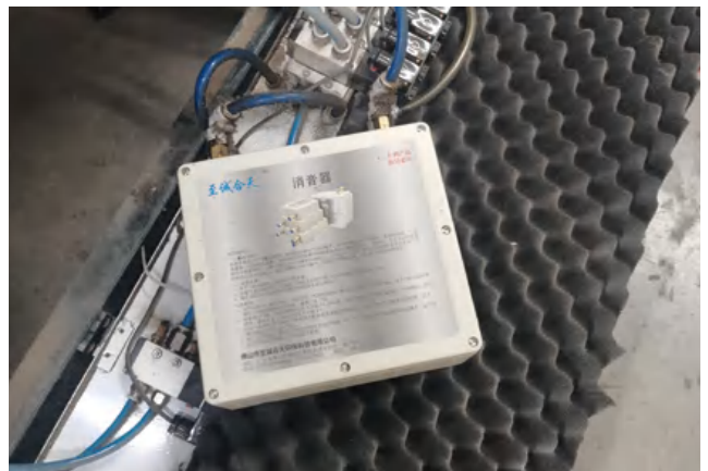
Silencers were installed to vacuum sound-emitting components
