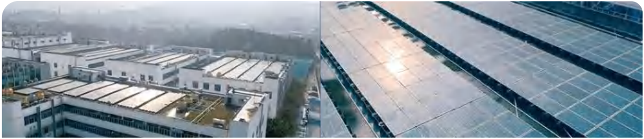
Solar Power Panels in Production Base
